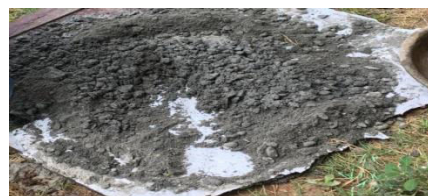
Fig: Concrete mixing
